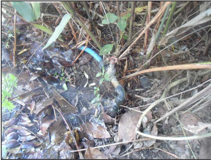
Close up of leaking pipe
